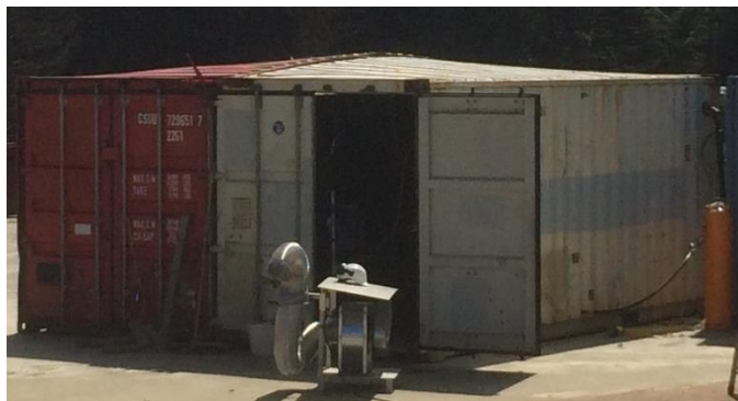
Figure 3.19: Ignition events deformed the roof of the test room and created a venting path.
