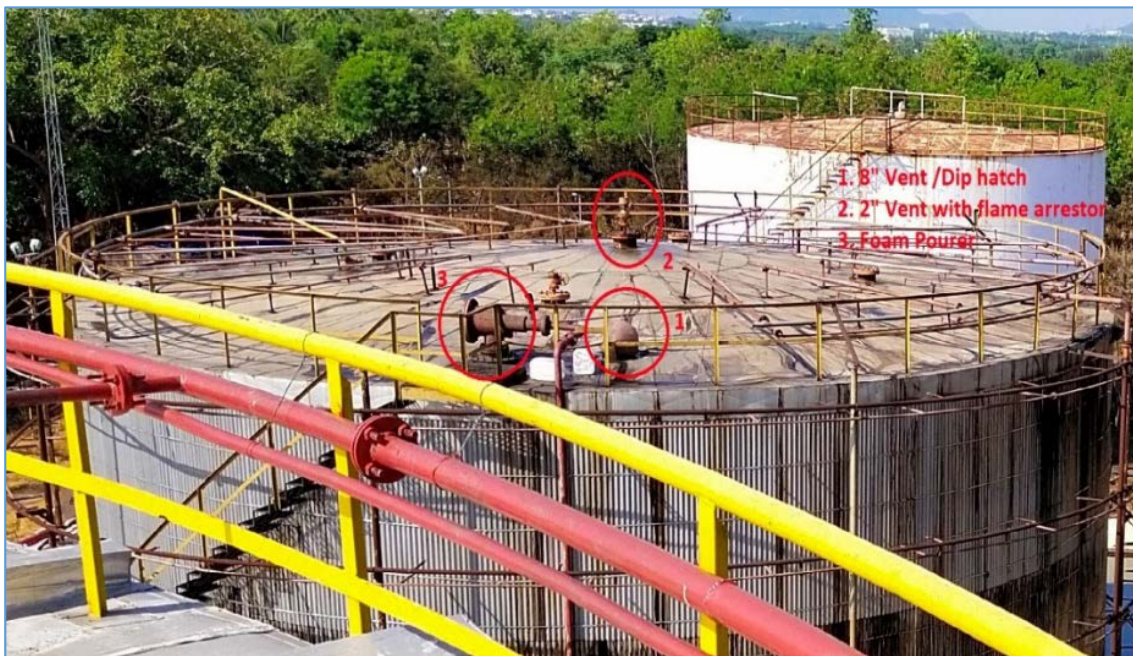
Figure 2.9: Roof Top of M6 Tank Showing Vents
