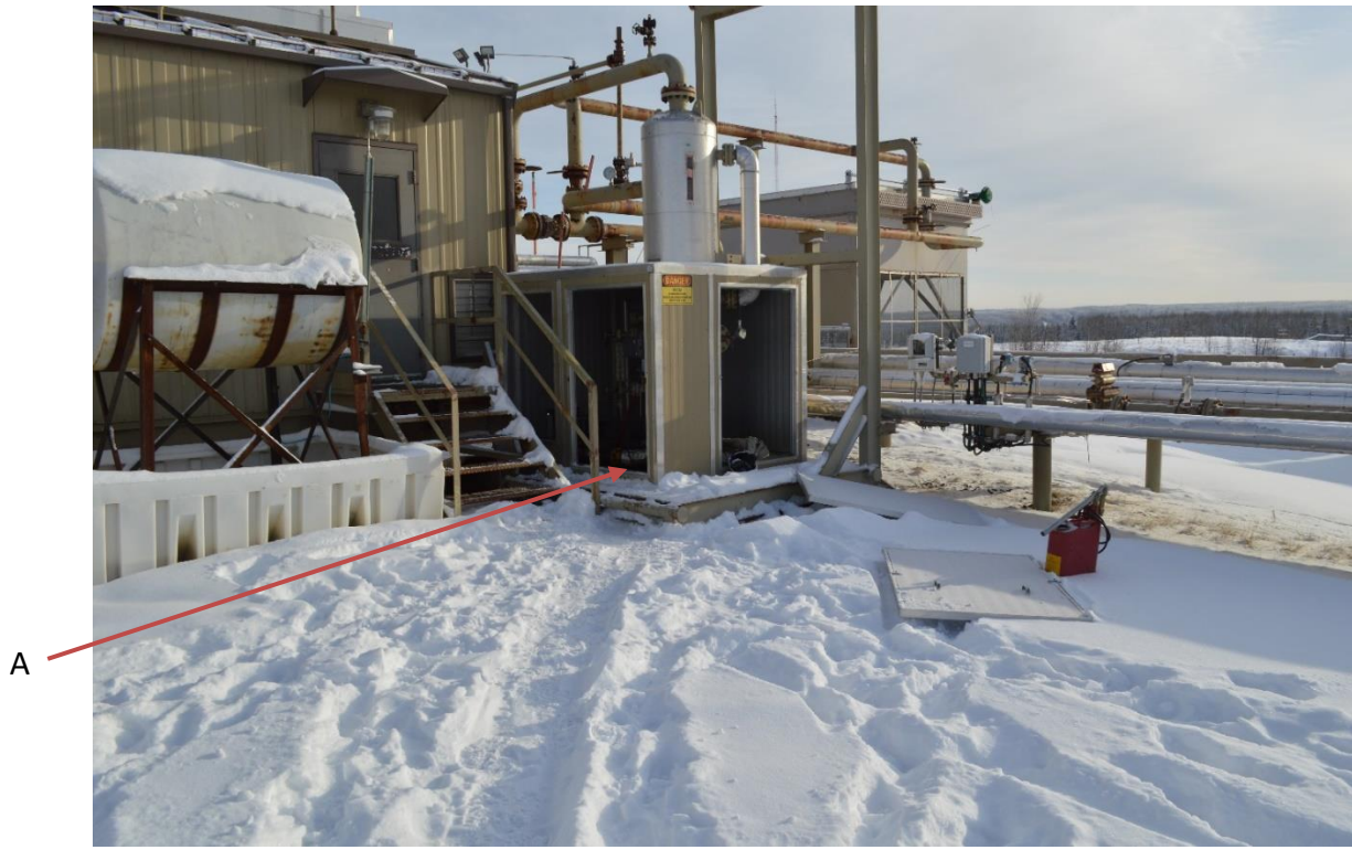
Figure 3. Door where Operator 2 first saw Operator 1 unresponsive partially inside the cyclone separator utilidor.
